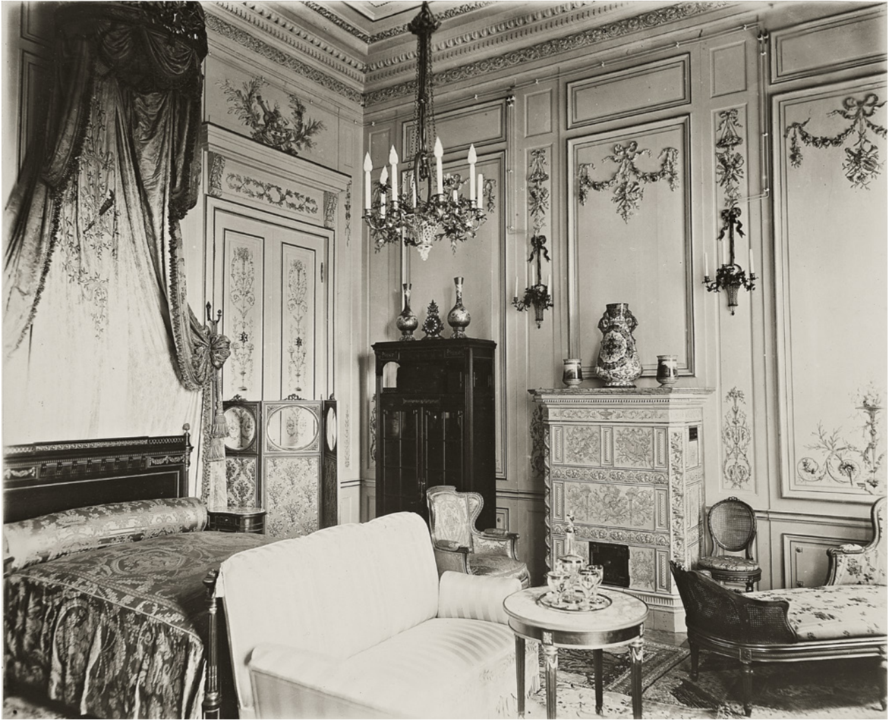
21 Küçük Mabeyn Pavilion Upper Floor Sultan's Room: Photographs of the buildings and gardens of the Yıldız Palace
